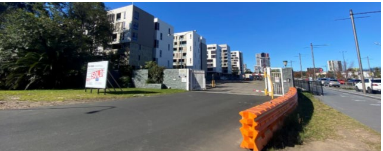
Figure 14 Developments to the north-west as viewed from Zetland Avenue (Note, Ausgrid site in foreground) (Source: Planning Ingenuity)
